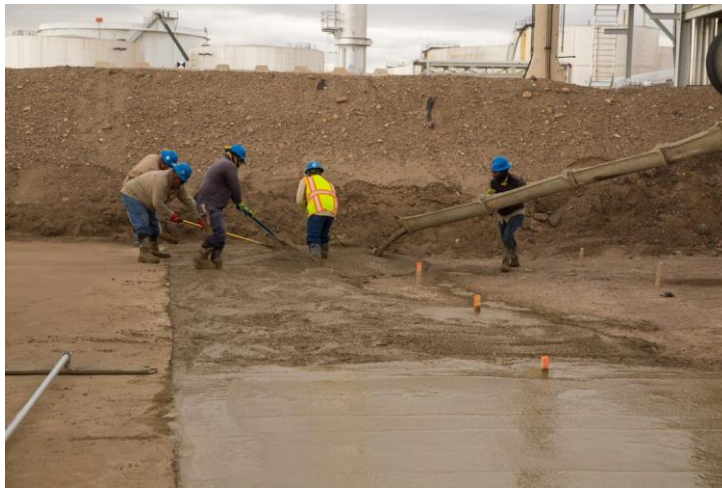
Pouring concrete for RD at Great Falls
