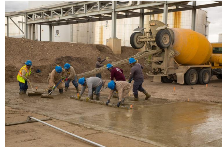
Leveling concrete for RD at Great Falls
